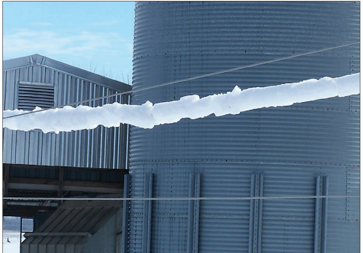
Ice and snow accumulated on power lines between five and six inches thick making restoration difficult.
