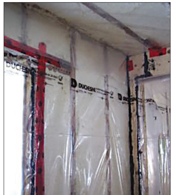
Right: Vapor barriers, like this plastic sheeting, trap moisture which causes mold.
