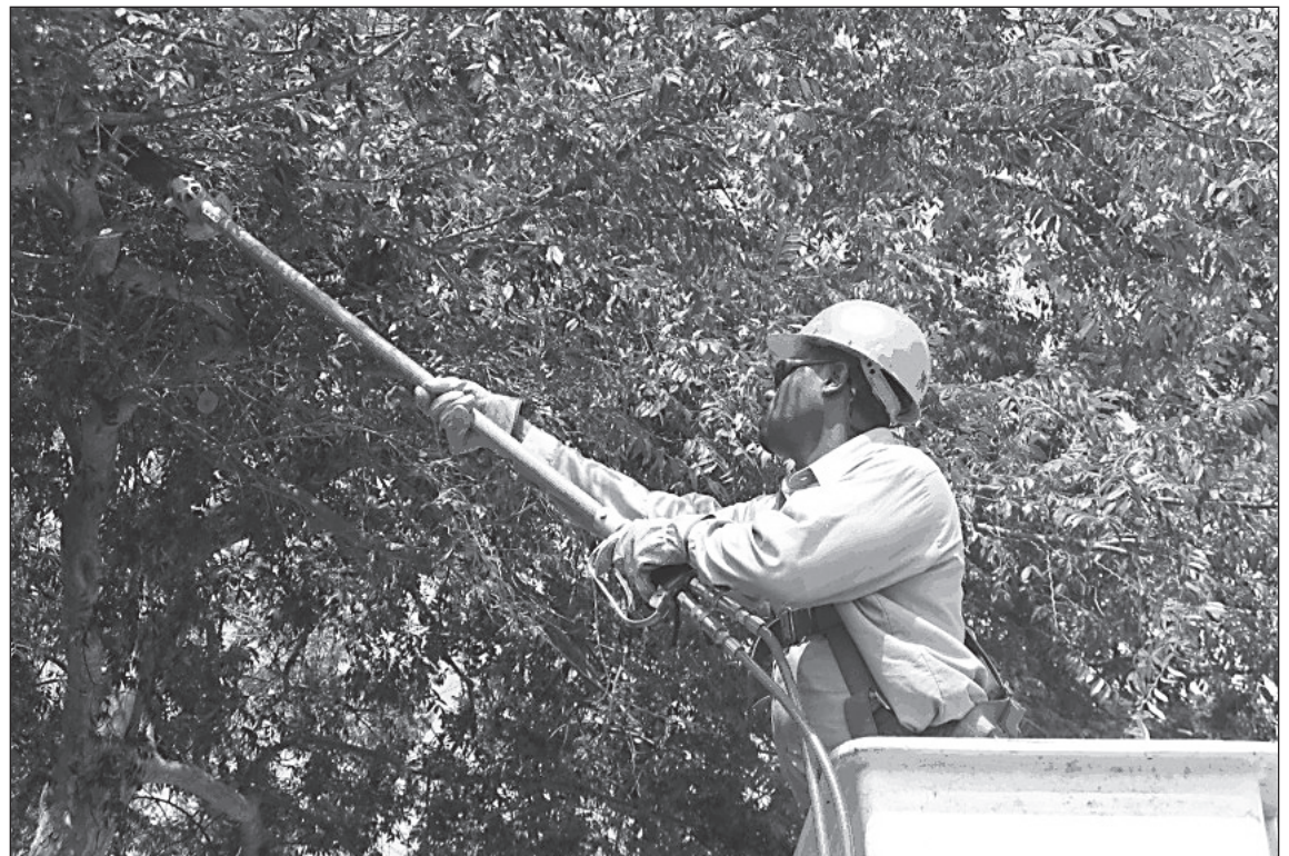
Electric utilities, like Miami-Cass REMC, trim trees for many reasons including safety and reliability. Trees are the leading cause of outages at Miami-Cass REMC.
